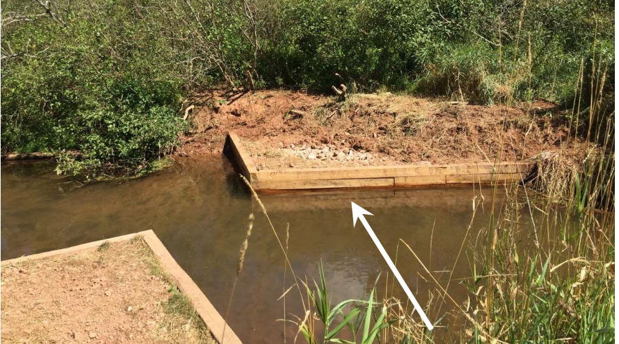
New wing deflector built to better “pinch” stream
