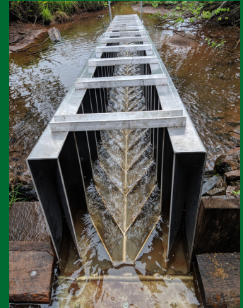
Looking downstream into a fish ladder
