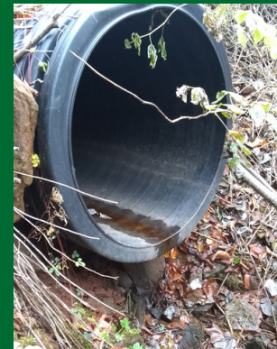
A hung culvert with very low flow
