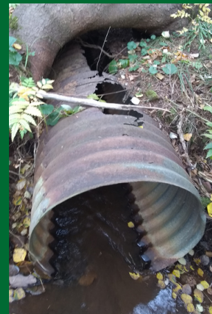
A rusted and decaying culvert
